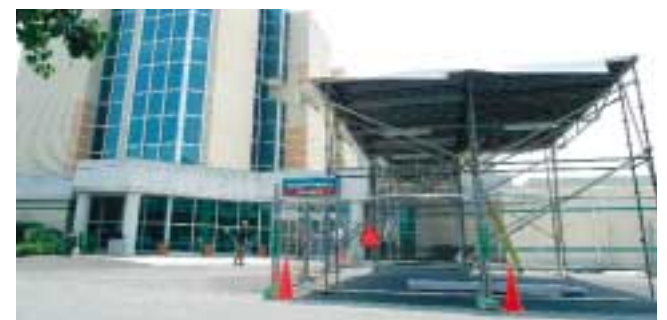
Emergency Department patients should use the East Entrance (above); all other visitors and patients are encouraged to use the West Entrance and park in the garage located behind the hospital.
